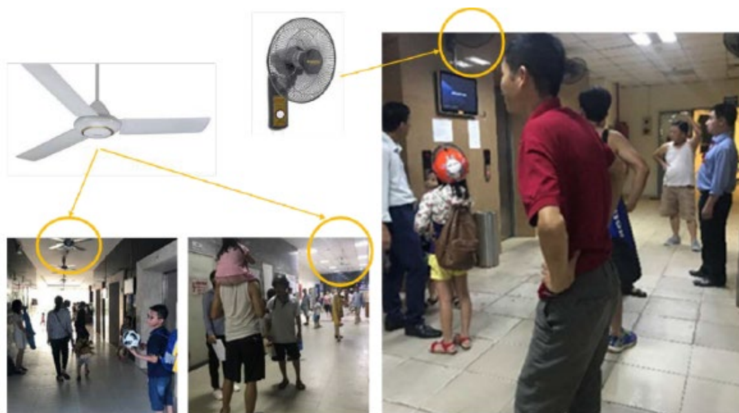
Figure 8. Lift lobbies on the ground floors (1) Kien Hung (2) Thanh Ha (3) Dai Thanh
